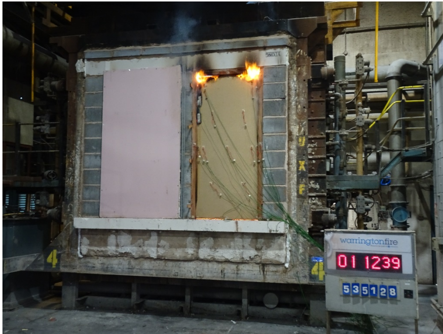
Figure 26 Unexposed face of Doorset B after 72 minutes of testing prior
